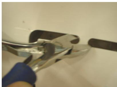
Snip perforated panel tabs
