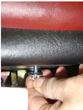
21. Install seat cushion. Add washers and hex nuts. Tighten nuts with small adjustable wrench.
