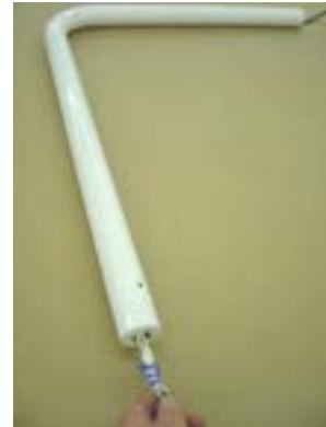
Gently pull wire harness connectors and wire harness from the bottom of the light post
