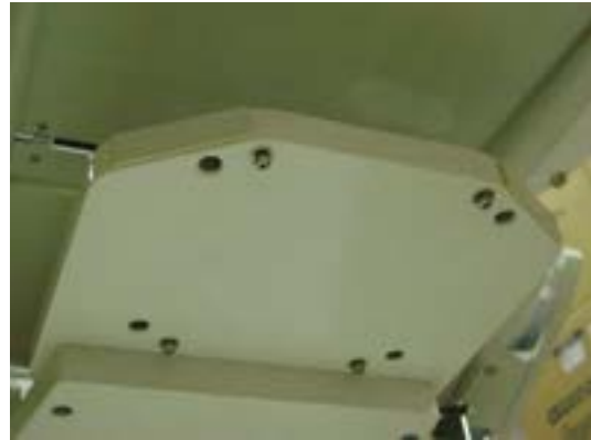
Attached mounting bracket, seen from below. Note (4) 4mm x 10mm Phillips screw heads face down. (These are used for mounting sensor/switch box for Clesta light )
