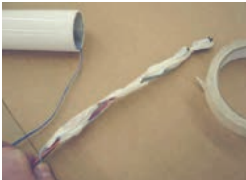
Tape the connectors at the end of the wire harness from the light in a loose helix with masking tape
