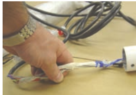
Wrap end of pull-string ribbon wire around taped connectors and insert into the Upper Curved Light Post at the end that has (2) holes
