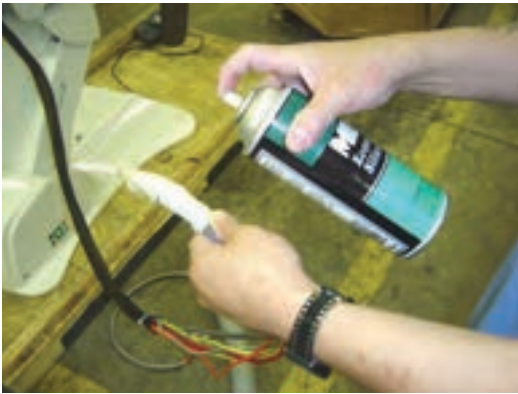
Apply a light coating of silicone spray to the outside of the tubing.
